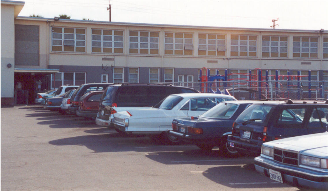
Figure 4: Main building east face
