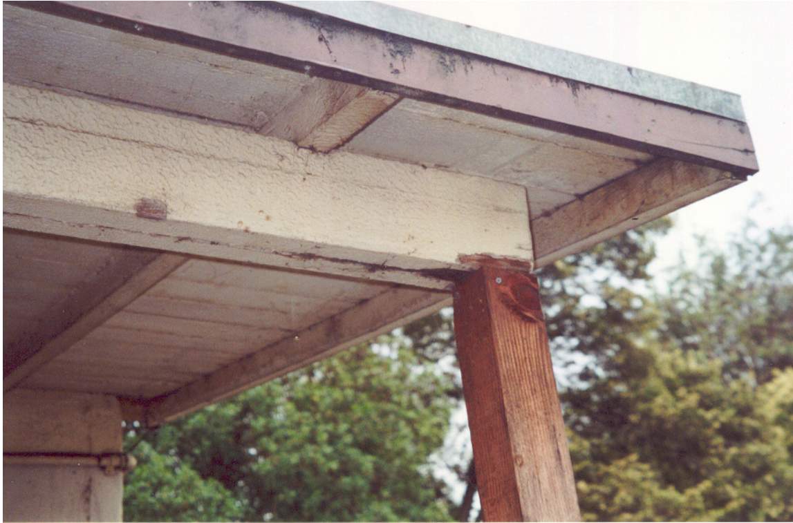
Figure 12: Deterioration of beam at classroom building covered walkway
