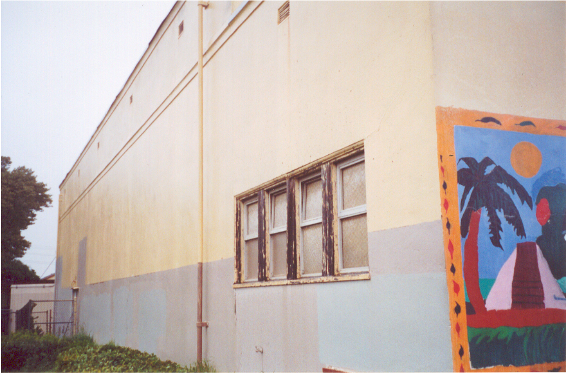
Figure 8: South face of cafeteria building
