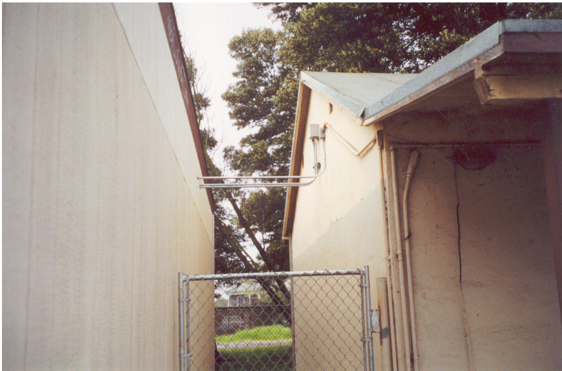
Figure 13: Conduit between cafeteria and classroom buildings
