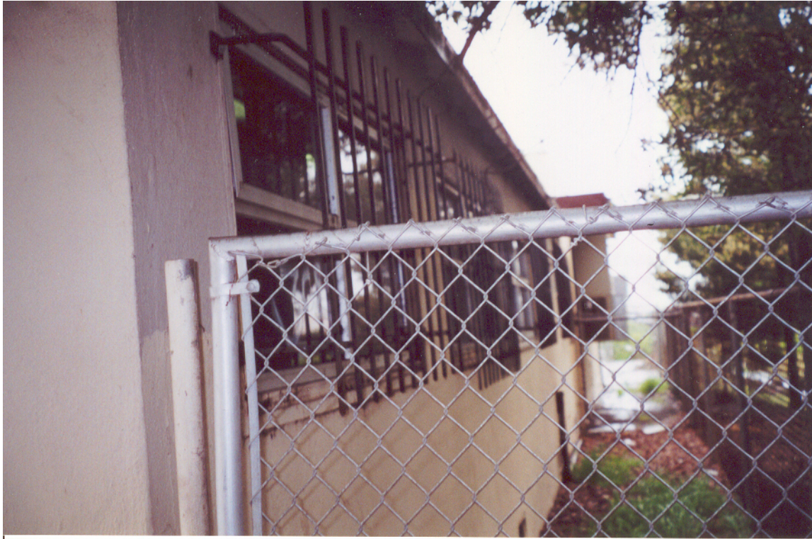
Figure 10: Rear face of classroom building
