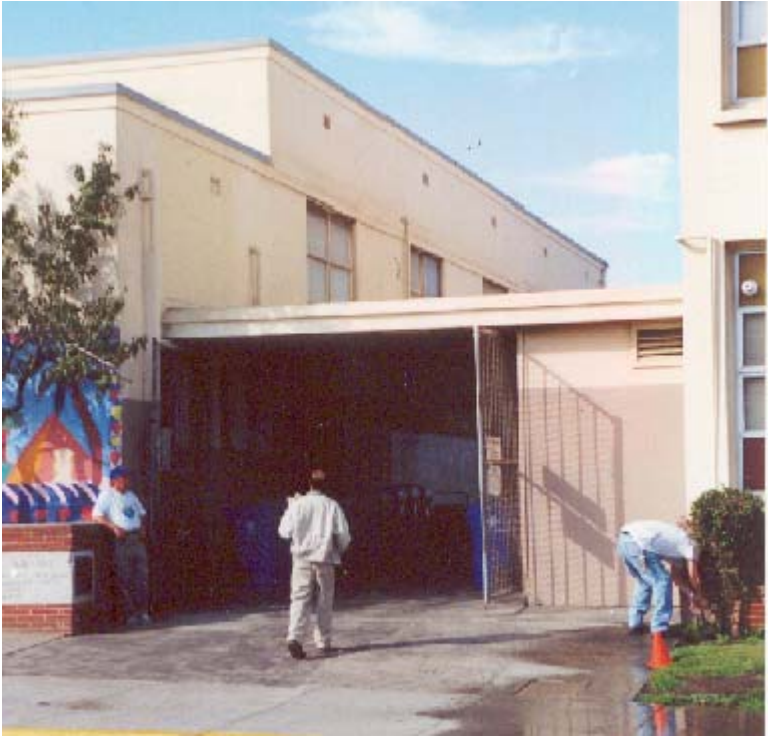
Figure 7: Covered walkway and cafeteria building north face
