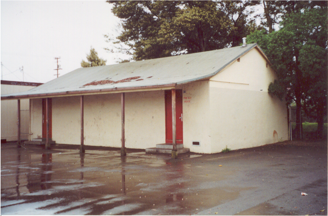
Figure 9: Front view of classroom building
